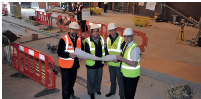
Work on the new 90 station Tone Zone is well under way at East Riding Leisure Beverley.
