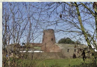
Former windmill by the old railway
